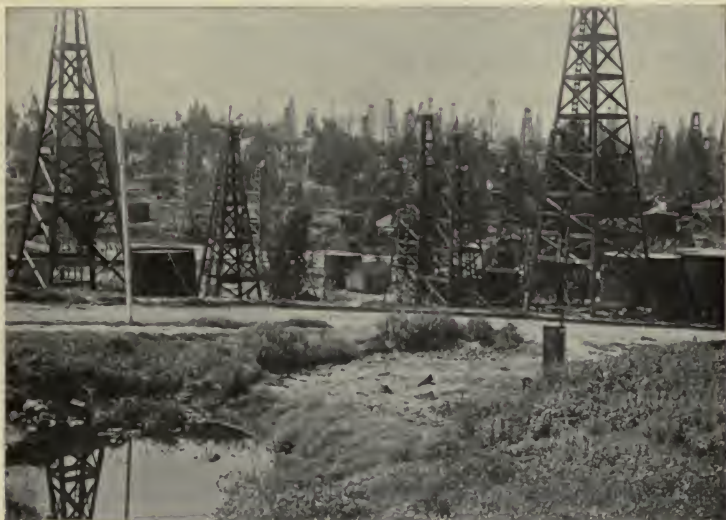
FIG. 110. — OIL WELLS IN THE CITY OF LOS ANGELES, CALIFORNIA Pool of oil in foreground
